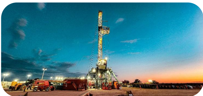
All lighting must be directed downward and contained to the site (Picture: Omega Oil and Gas)
