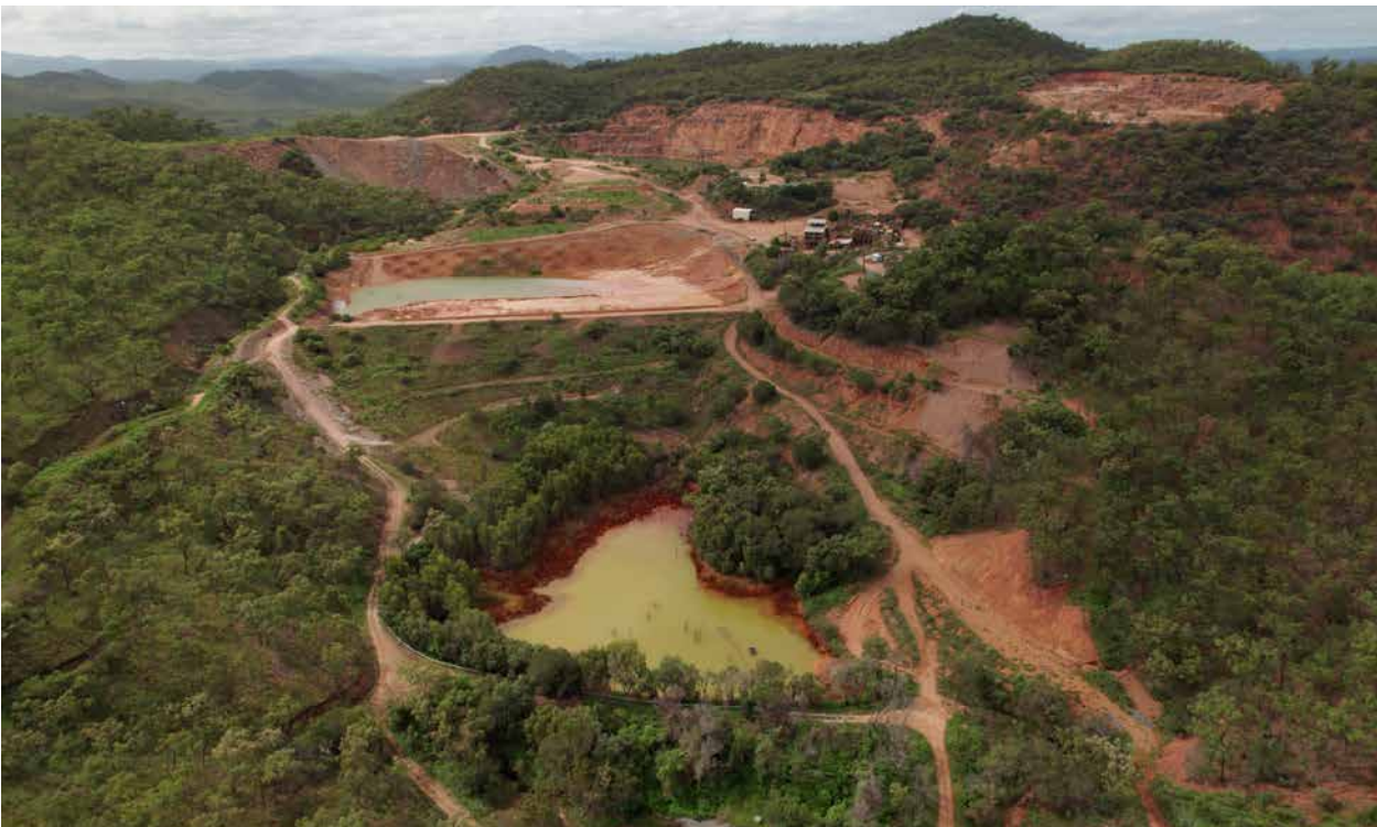
Wolfram Camp tailings dam
